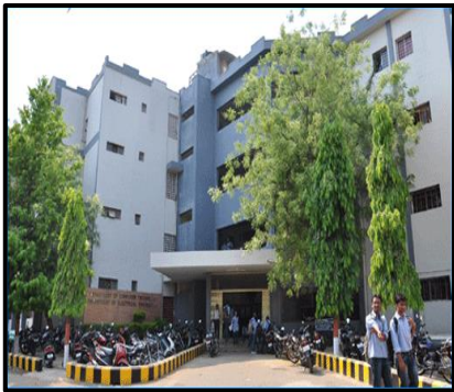
Computer & Electrical Block
